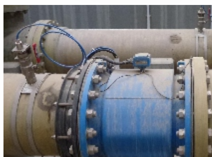
Installation of ultrasonic flow measurement using NFP
