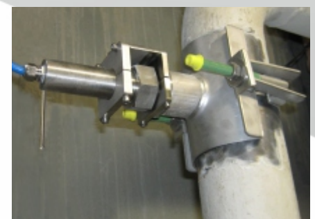
Installation of ultrasonic flow measurement using NFP
